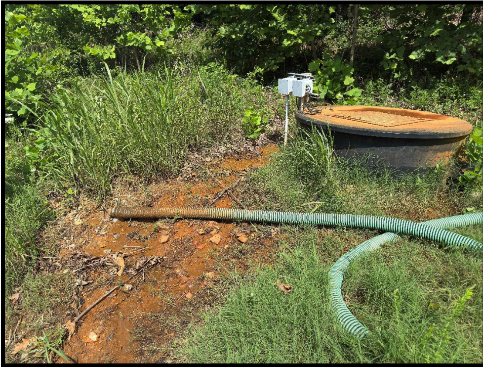
Photograph 1: View of erosional rill from VLCS-1 overflow.
